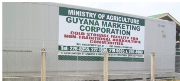
Figure 20 (e): One of the Refrigerated Containers found at the Packaging Facilities
